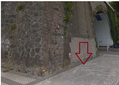
P05: Ondarreta Tunela
